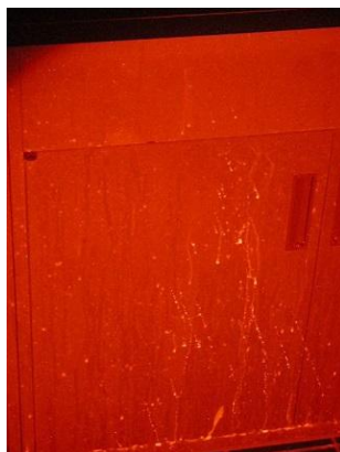
cabinet under sink; CSS, Orange Filter
